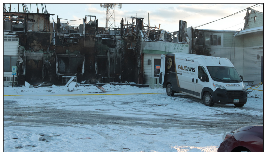
Superior & Sage Hotel's front door with Paul Davis Restoration van parked outside on Feb. 24.
