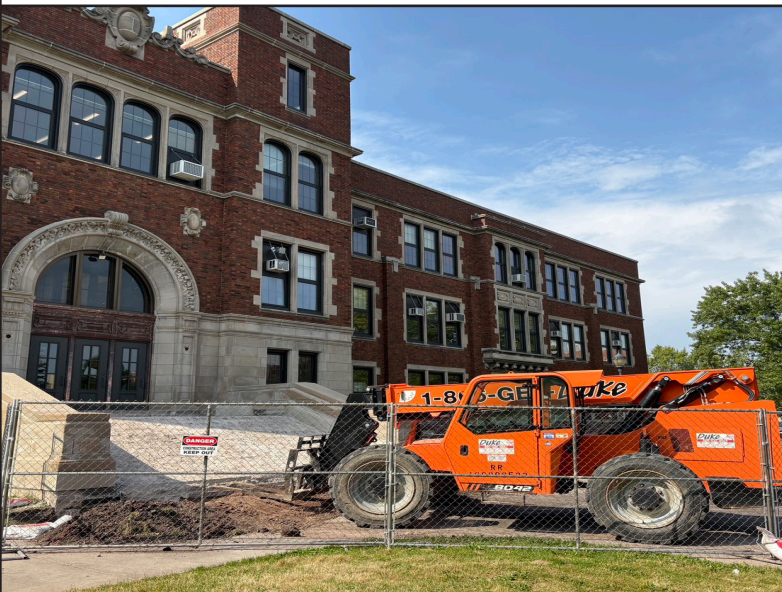
Restoration of Old Main stairs on Sept. 15, 2025.
